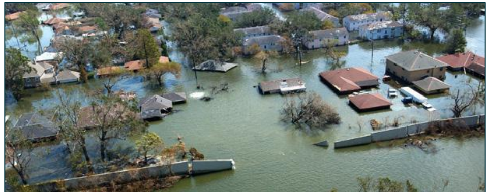
Figure 8. Flood: the problem of excess water.
