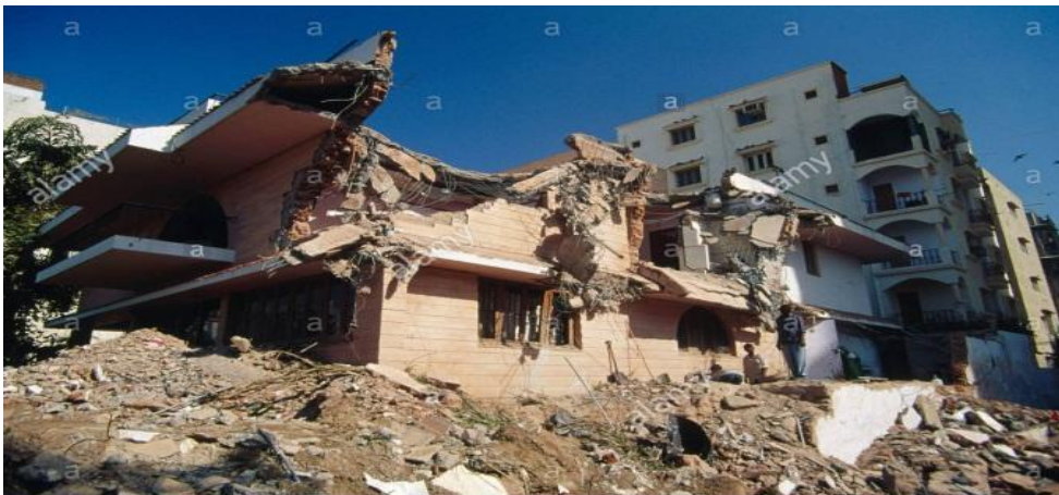
Figure 05: Destruction caused by Bhuj Earthquake.
